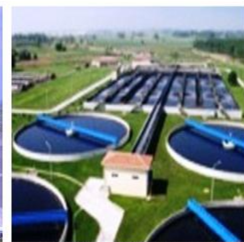
BESLER GIDA WASTEWATER TREATMENT
